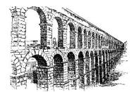
aqueducts, or waterways. These under and aboveground channels, typically made of stone, brick, and volcanic cement, brought fresh water for drinking and bathing as much as 50 to 60 miles from springs or rivers. Aqueducts helped keep Romans healthy by carrying away used water and waste, and they also took water to farms for irrigation. So how did aqueducts work? The engineers who designed them used gravity to keep the water moving. If the channel was too steep, water would
